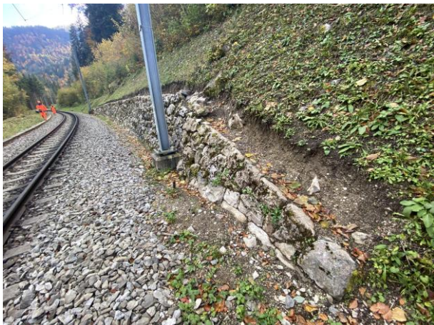
Figure 1 : KM 24.425 - Mur existant amont
