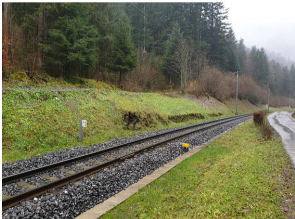
Figure 28 : KM 26.174 - Mur existant amont
