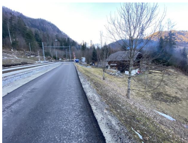
Figure 10 : KM 24.980 – Route du Revers direction Montbovon
