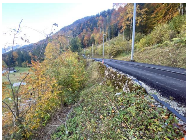
Figure 23 : KM 25.140 – Mur aval
