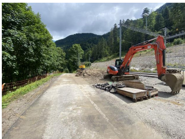
Figure 11 : KM 24.990 – Route du Revers direction Rossinière
